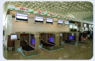
With a rise in passenger numbers and an increasing need for check-in counters, CSMIA took the approach to add 25 SBD's [incremental capacity]. It helps passenger to be self-sufficient for check in of their baggage leading to a 12% incremental capacity addition at the check-in processor.
